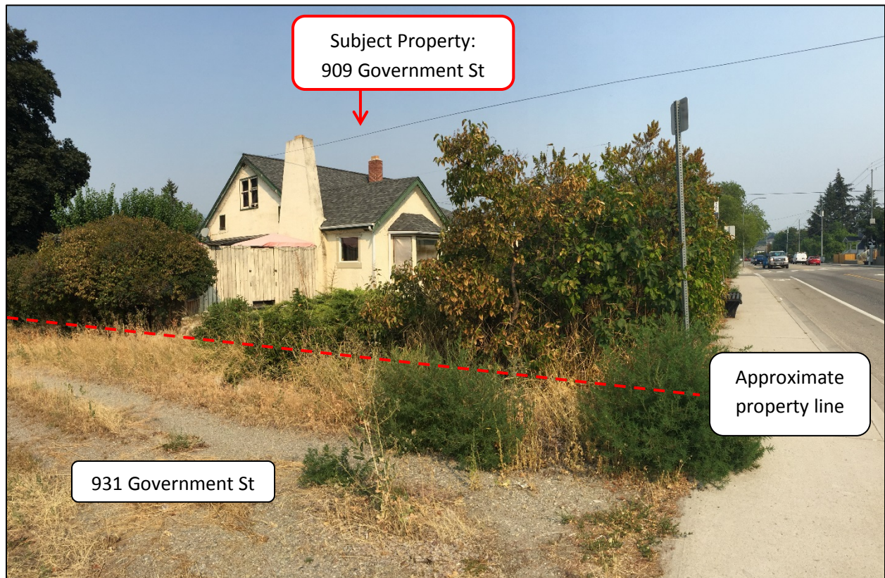
Figure 6 - Looking at 909 Government St from Government St (looking north)
